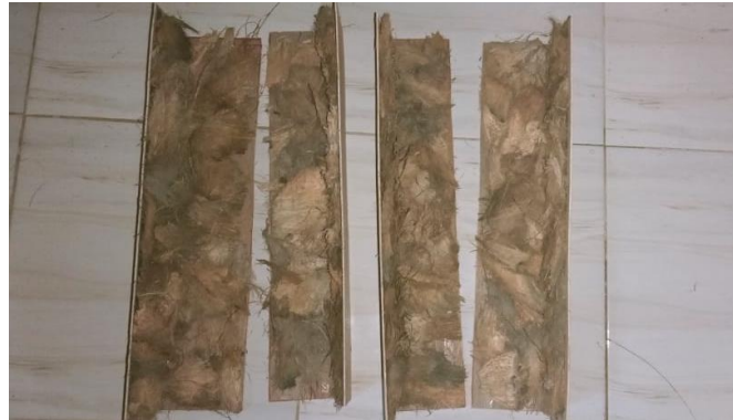
Figure 4. Installing coconut fiber on a plywood board
